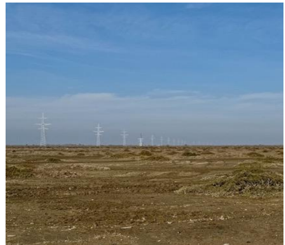
Newly installed OHL towers at Banka, going towards Navahi
