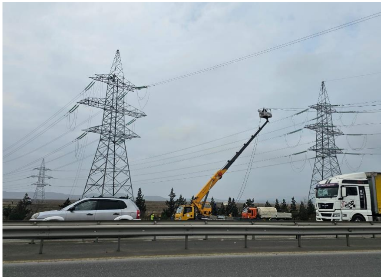
Newly installed OHL towers at Baku-Gazakh highway encroachment, going towards Navahi
