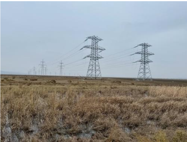
Newly installed OHL Towers at Navahi, towards Banka and Bilasuvar
